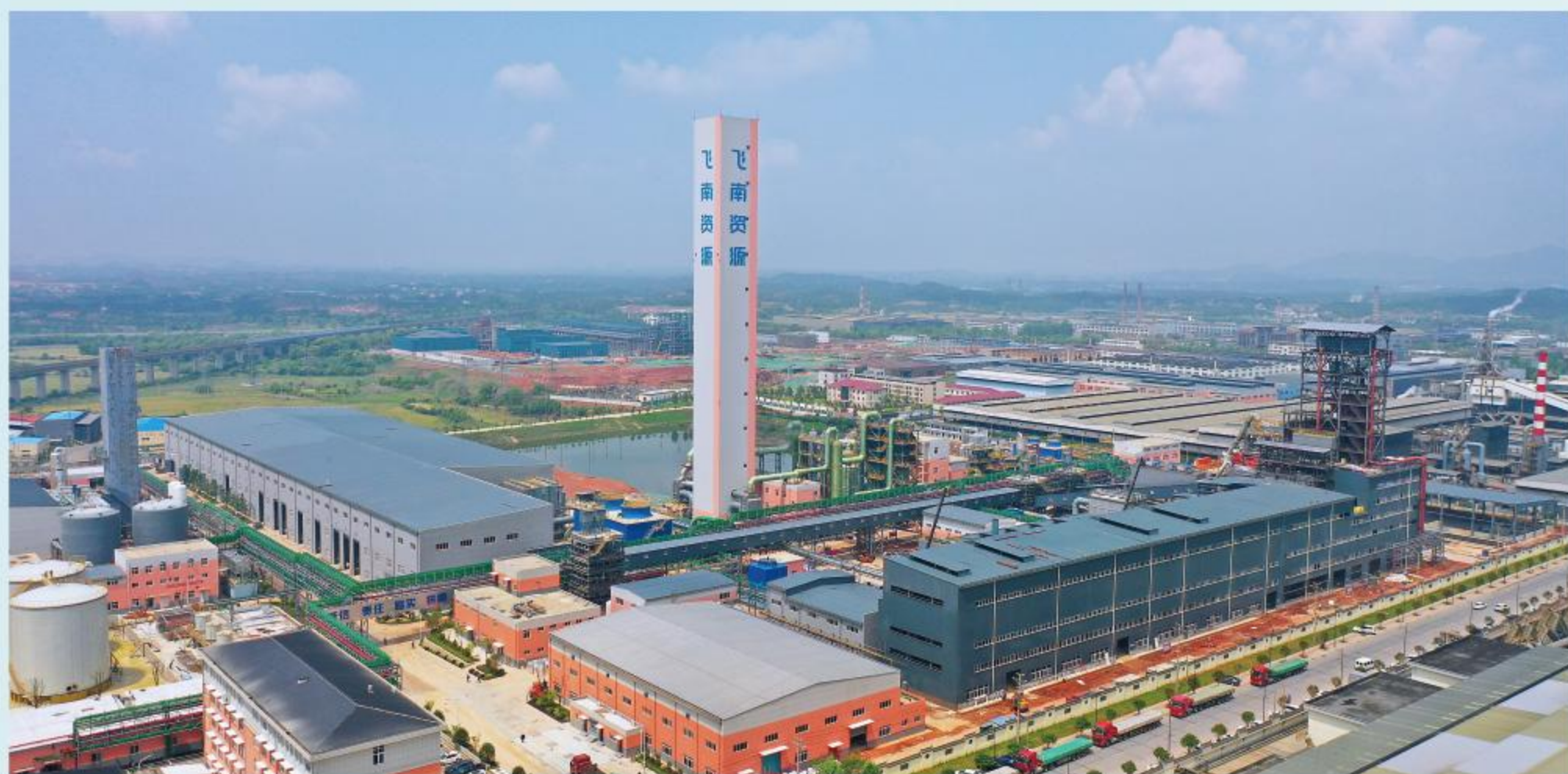
江西南危固废处置项目 Project of Hazardous Solid Waste Treatment for Jiangxi Xingnan Environmental Protection Technology Co., Ltd.
